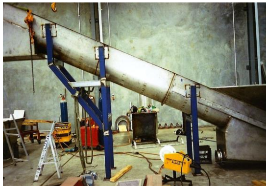
Classifier Fabrication at Malaga Workshop VOR Environmental
